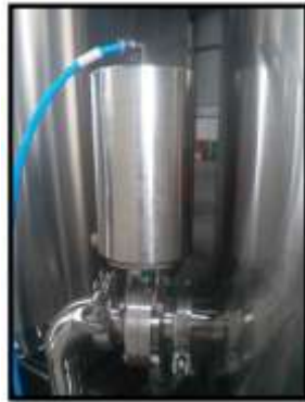
Gambar 1. Butterfly Valve Pneumatic.
