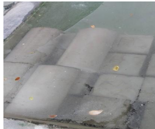
Gambar 7. Proses Perawatan ( Curing ) Beton
